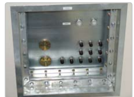
Penetration panel with C-type frame
