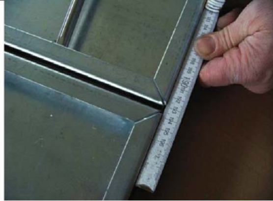
12. Before bolting together, the modules have to be aligned
