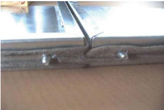
7. The mesh must overlap
