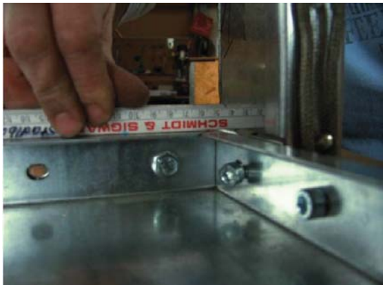
13. Before bolted together, the modules have to be aligned
