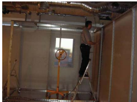
16. Start installation of the ceiling
