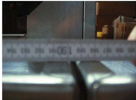
14. Before bolted together, the modules have to be aligned
