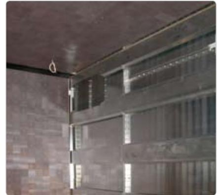
Structure for the installation of ferrite absorbers
